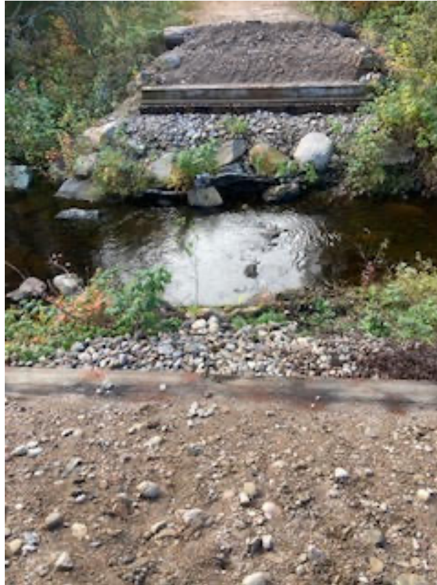
Winter crossing decommissioned to avoid sedimentation
